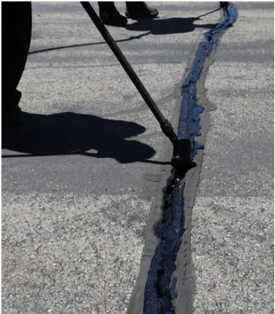
Crack Sealing
