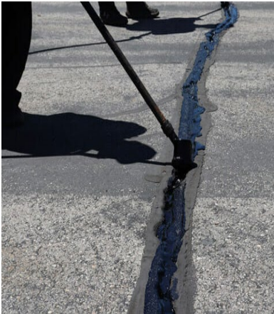
Crack Sealing
