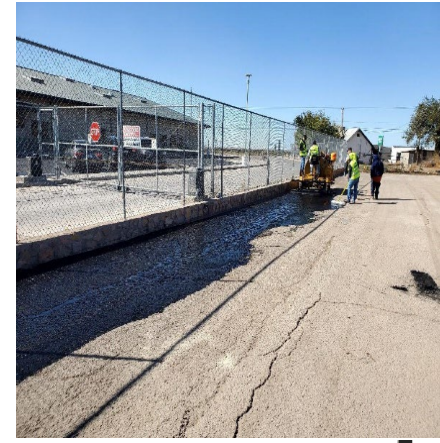
Slurry Sealing
