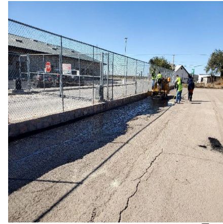
Slurry Sealing
